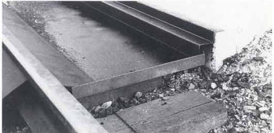
*On this installation, concrete platforms were poured with a nosing angle on the edge. A zee flashing angle is welded to the angle, protecting against oil leakage.*
