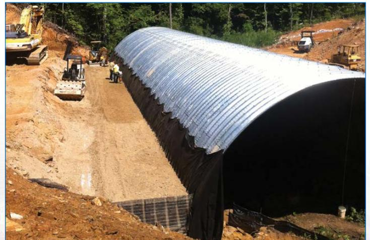
35'-8" x 17'-10" BridgeCor Backfill with Welded Wirewall – Gainesville, Georgia
