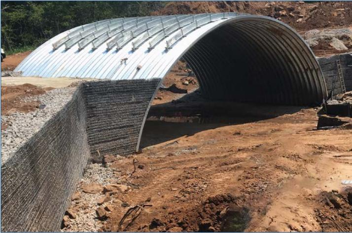
BridgeCor External Rib System ( 64'-2" x 19'-7" ) during construction
