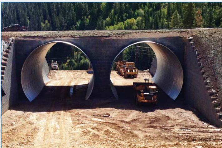
(2) 50' Round BridgeCor structures provides a variety of sizes for buried inverts necessary in grade separations needed for mine access roads and tunnel entrances.
