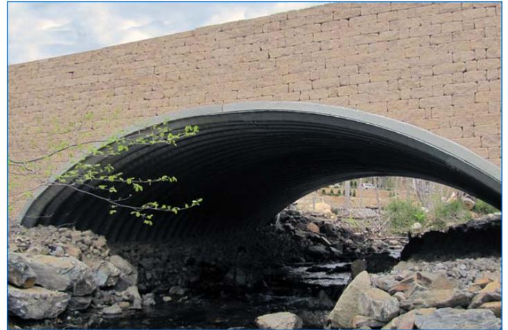
21'-2" x 10'-8" BridgeCor Arch with Keystone® Retaining Wall Systems - Shelton, Connecticut
