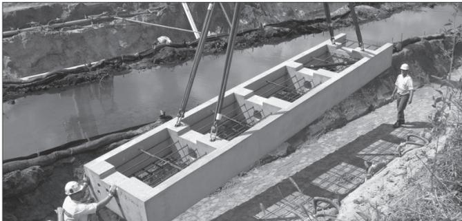
1. Attach foundation segment to the crane using preset lifting inserts in the precast foundation at all four locations. Slowly lower in to place taking care to line up correctly with the layout in Step I.
