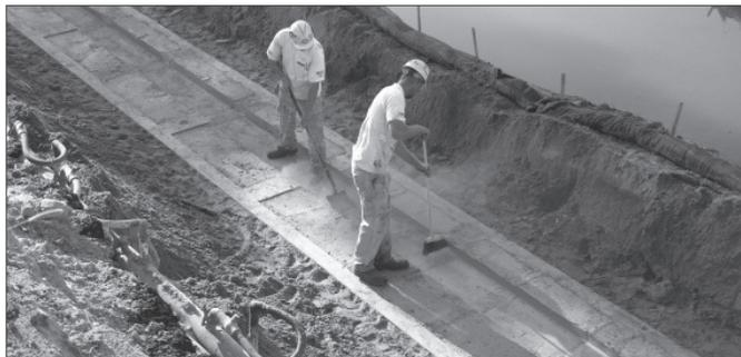
4. Once infill concrete is set, strip keyway forms and sweep clean.
