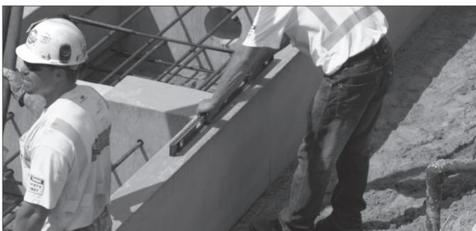
2. Check to make sure the segment is either level or sloped according to the elevation points in the construction drawings. Variations should not exceed 1/4" per ten feet. Place the subsequent adjoining foundation segments in the same fashion.
