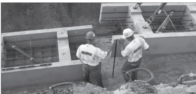
3. Match up connection at line and grade with the previous set segment making sure to leave 1/2" gap between segments per construction drawings.
