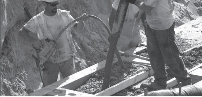
1. Block out vertical side of keyway using the proper size lumber to retain concrete infill and maintain the dimension of the keyway throughout the length of the foundation.
