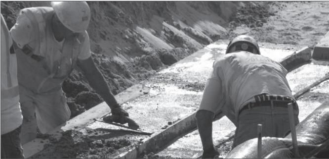
2. Pour infill concrete to top of foundation unit in each cell. Be sure to vibrate to consolidate mix and remove any voids.
