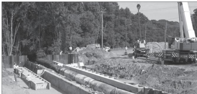
**II. THE TIME OF THIS CONCRETE POUR WILL IMPACT WHETHER A GROUTING STEP IS NEEDED. THE CAST-IN-PLACE CONCRETE CAN BE POURED PRIOR TO SETTING THE STRUCTURE OR AFTER SETTING THE STRUCTURE.**
