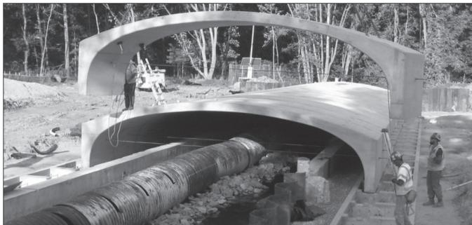
1. Once EXPRESS Foundations are set the entire structure, complete with arch units, headwalls and wingwall, is to be installed (for the structure installation refer to *Precast Bridge Installation Guide*).
