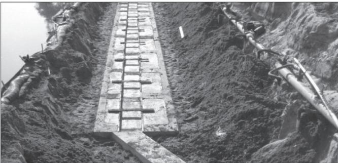
3. Float off concrete level with the top of foundation maintaining a level keyway. If applicable pour wingwall closure joints.
