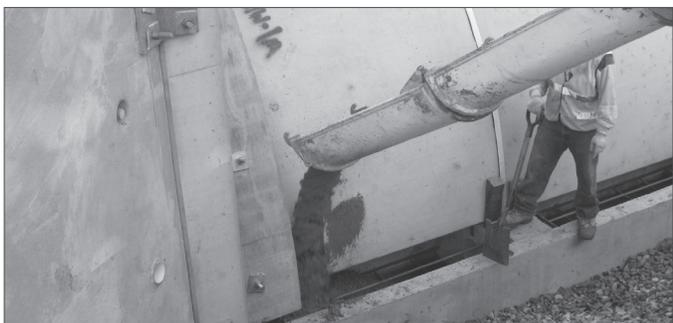
2. Once the entire structure is installed, the foundation concrete infill can be poured, vibrated and floated to the top of foundation segments.
