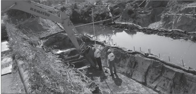
1. Excavate to the specifications in the construction documents. It is best to overexcavate the width a minimum 2' larger than the EXPRESS Foundation unit. In some cases a dense graded granular base material is specified as the leveling pad. Be sure to grade receiving pad +/- 1".
