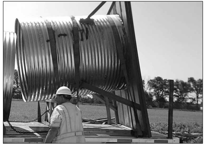
Lifting Aluminized Type 2 (ALT2) CMP with nylon slings.
