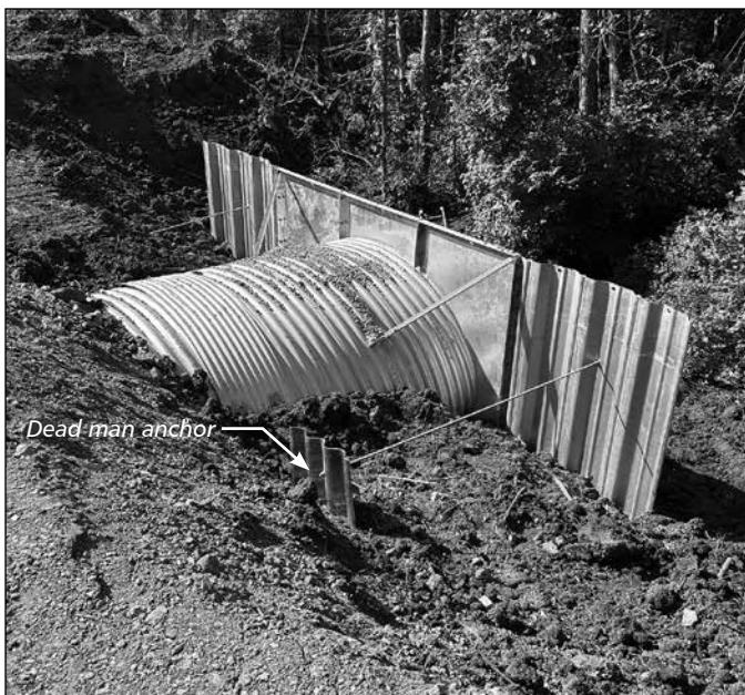
Threaded tie rods are bundled with metric sheeting.
