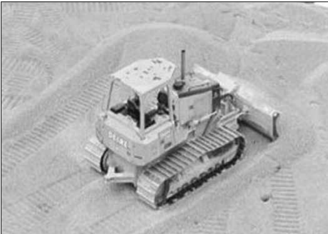
Examples of light, tracked, construction equipment used to place final cover over the pipe system. Keep a minimum of 12" of cover over the pipe prior to operating lightweight track equipment. Additional minimum cover maybe required for larger equipment.
