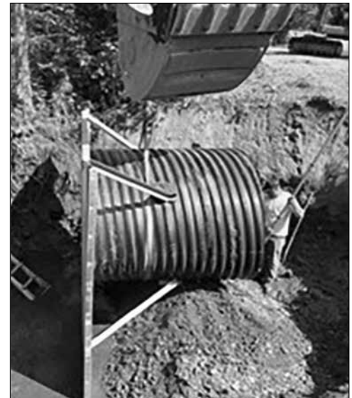
Lifting Aluminized Type 2 (ALT2) CMP with nylon slings.
