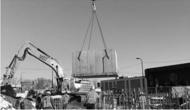
The contractor **MUST** provide all rigging and lifting apparatus, such as all cables, chains or straps and a set of lifting hooks, shackles, knuckles and eye bolts.
