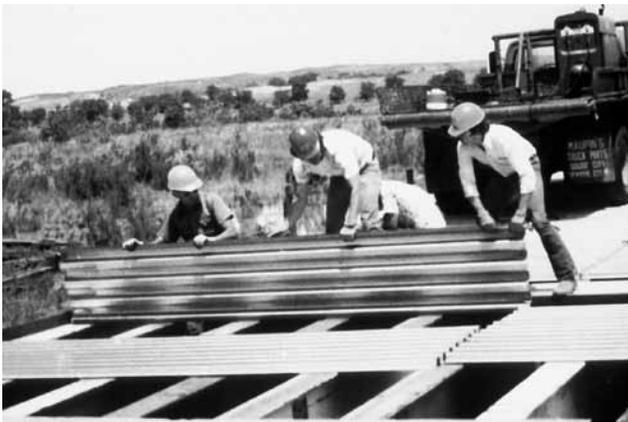
Contech Bridge Plank is installed quickly, at low cost.
